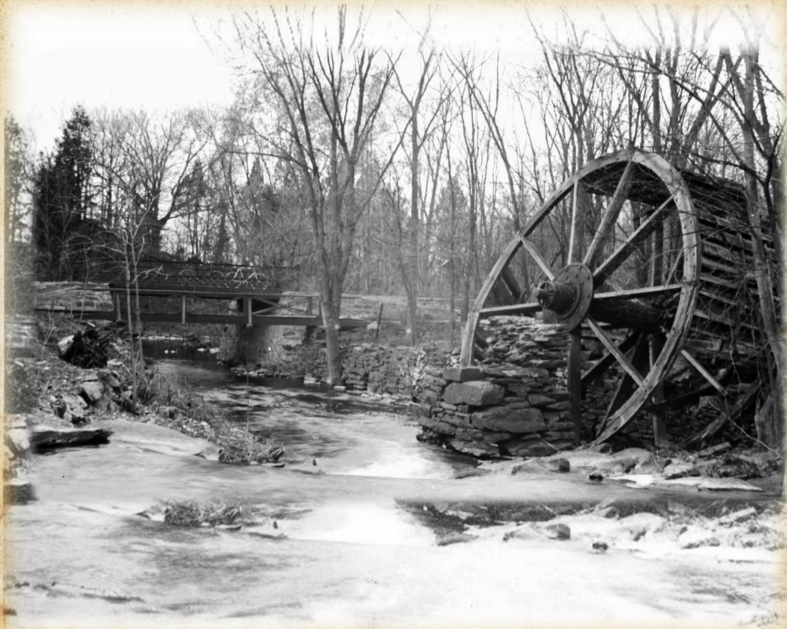
RM.1999.1101. Note: the current footbridge uses the iron rails from this old cart bridge (footbridge built circa 1912)
